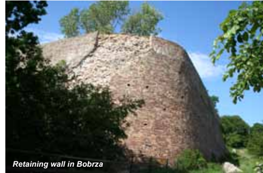
Retaining wall in Bobrza
